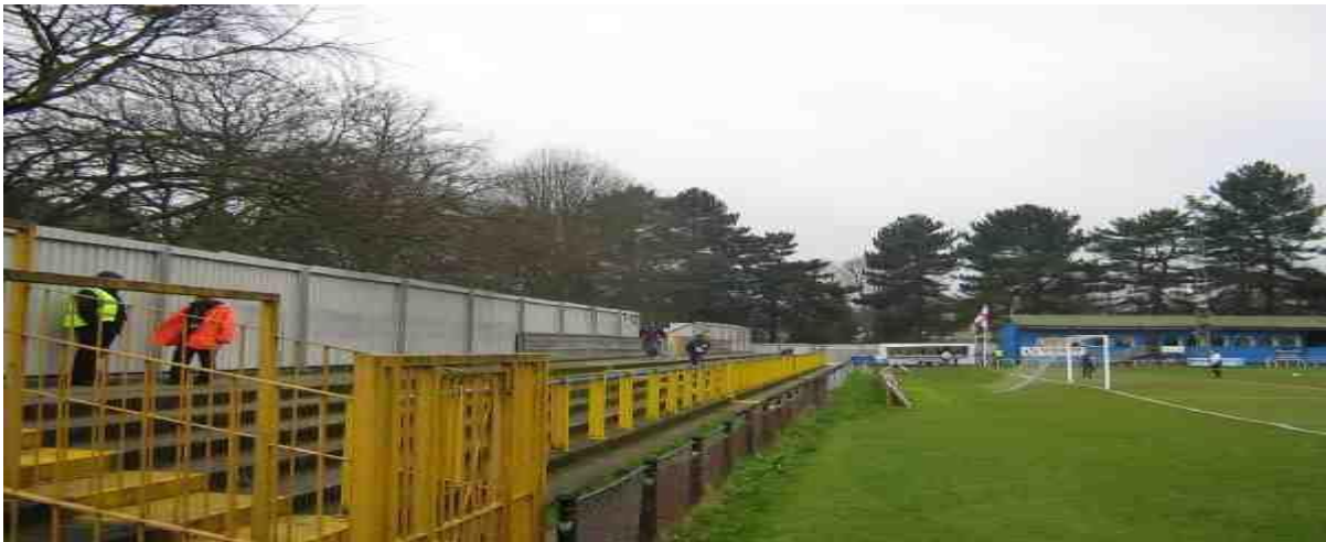
Hatfield Road of East Terrace
